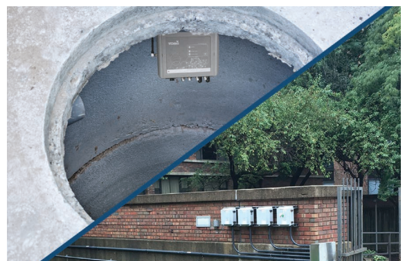
Monitoring/Alarm unit can be mounted inside or externally mounted (remote monitoring)
